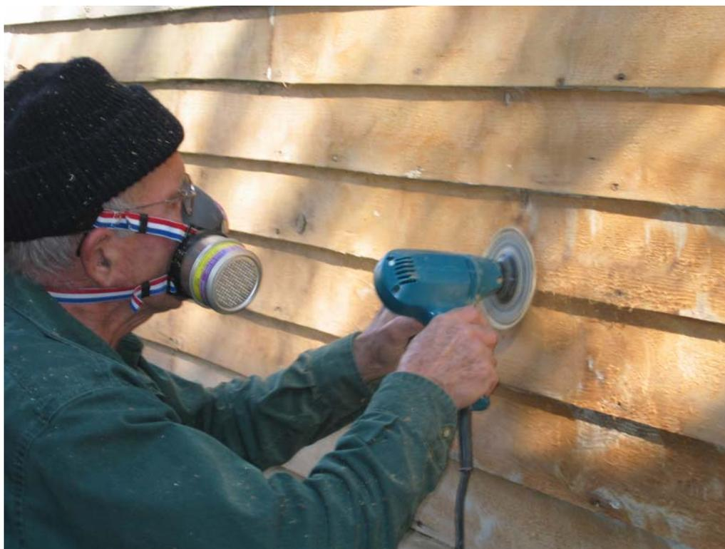
Sanding the surface following the Paint Shaver to remove small residuals of paint and to smooth the surface prior to treatment with water repellent preservative.
