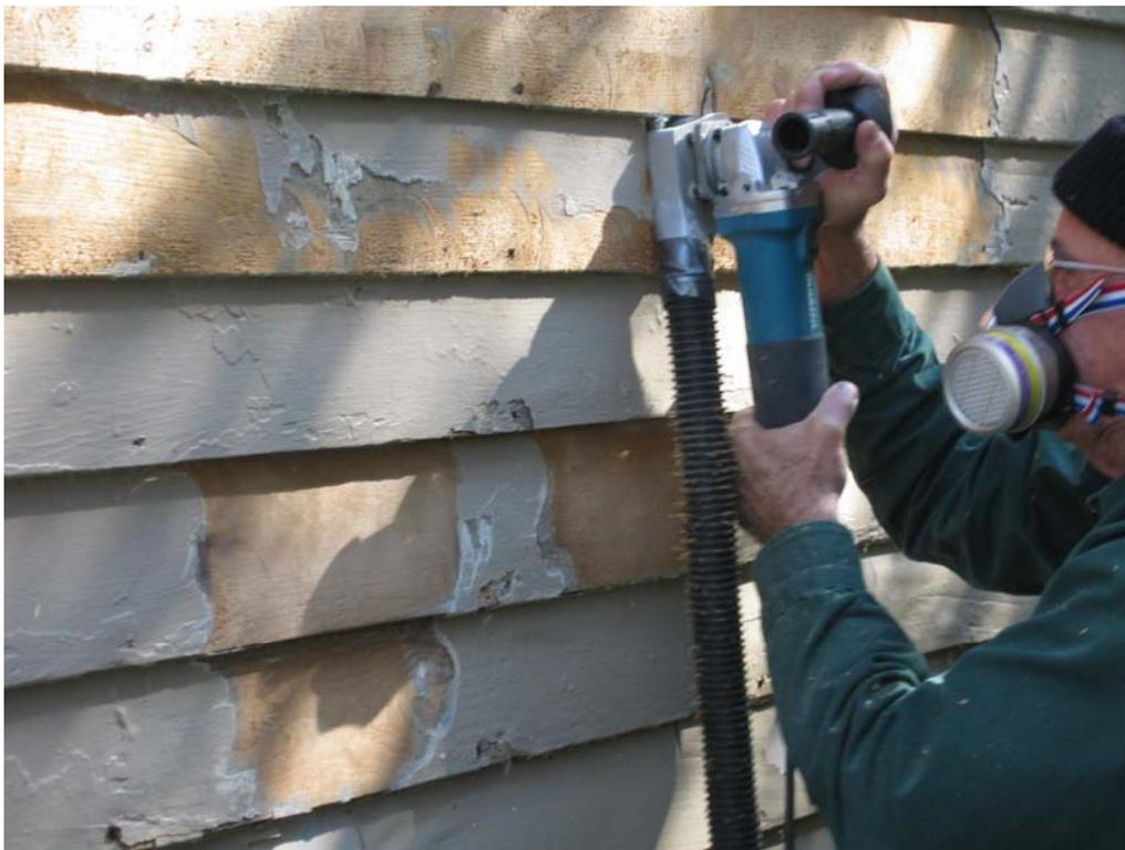
Removing paint with the Paint Shaver. The hose is connected to a vacuum, preferably a HEPA Vac, to collect lead paint chips and dust. Note operator is wearing respirator with lead filters to protect against lead dust.
