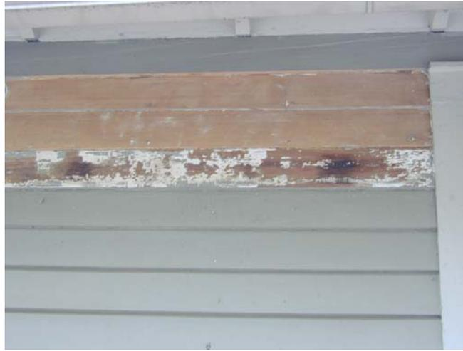
Appearance of Top Group after paint removal by Paint Shaver, hand scapping, and Silent Paint Remover, in that order from top to bottom.
