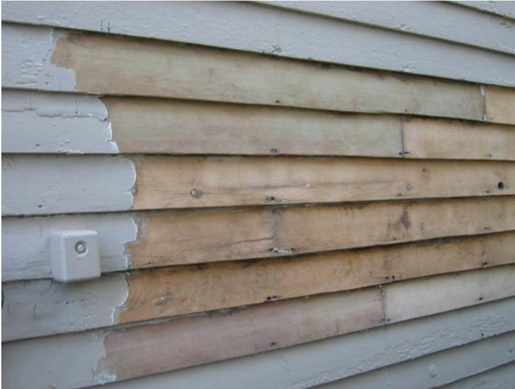
Surface ready for water repellent preservative treatment, filling of holes and painting after paint stripping by Paint Shaver followed by light sanding. Note the edge of the area of remaining paint. It indicates heavy, hard paint.
