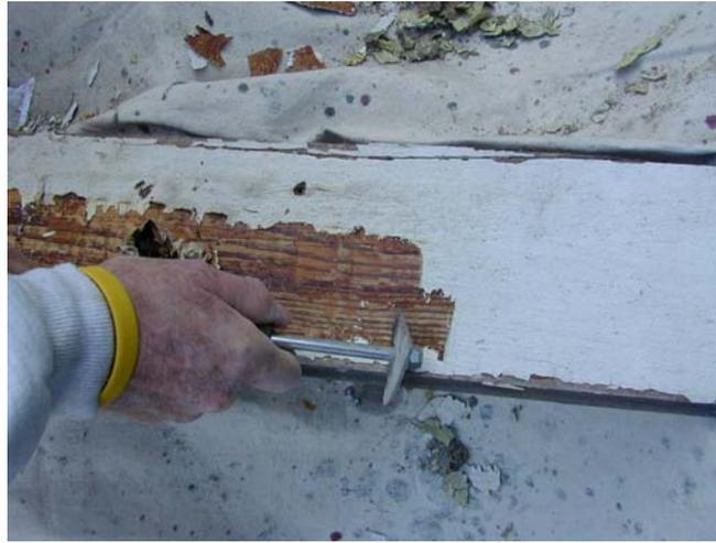
Paint softened by Silent Paint Remover is easily and completely scrapped from a painted board
