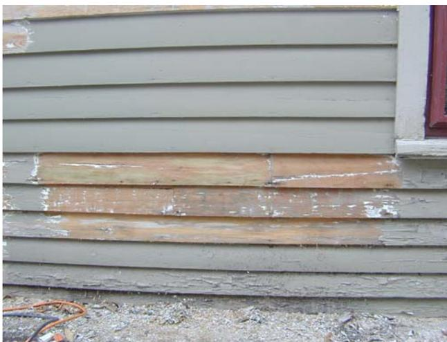
Appearance of Bottom Group after paint removal. Paint Shaver, hand scrapping, and Silent Paint Remover, in that order from top to bottom.
