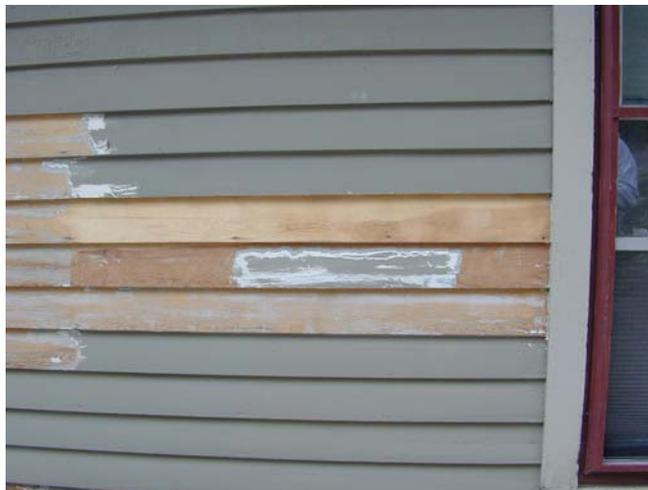
Appearance of Middle Group after paint removal. Paint Shaver, hand scrapping, and Silent Paint Remover, in that order from top to bottom.
