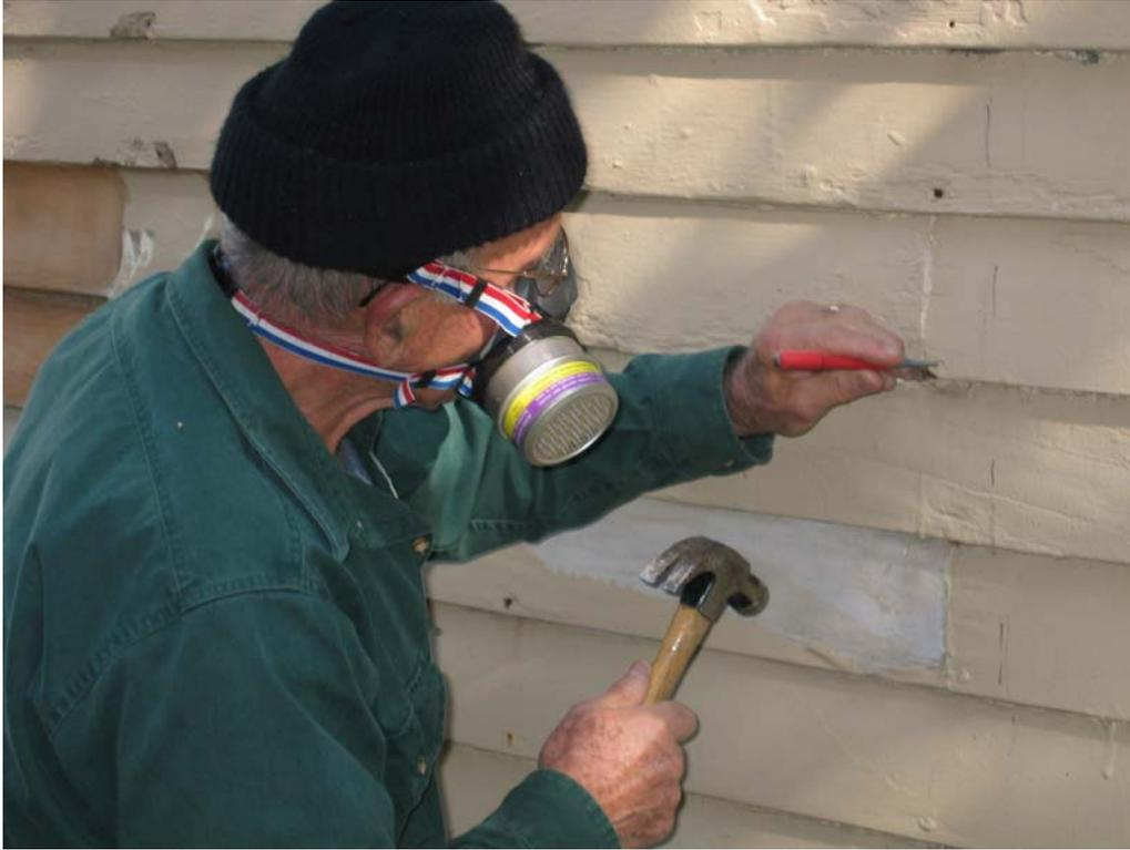
Setting nails prior to removing paint with the Paint Shaver<sup>®</sup>
