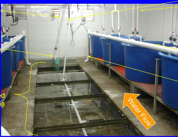
Air Lines to Tanks and Filter
