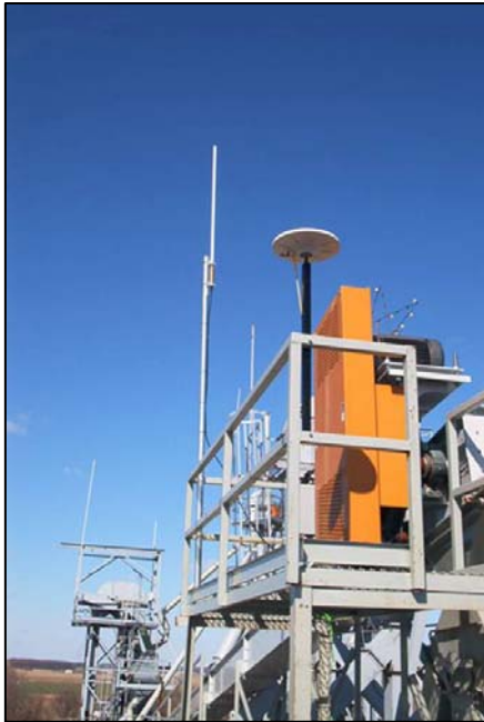
This Tri-State RTK base station, consisting of a control box, RTK base, and radio antenna is located on top of an Ohio grain elevator.
