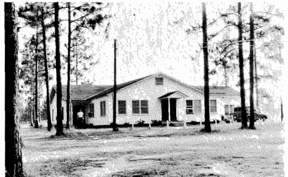
The air conditioned mess hall.
