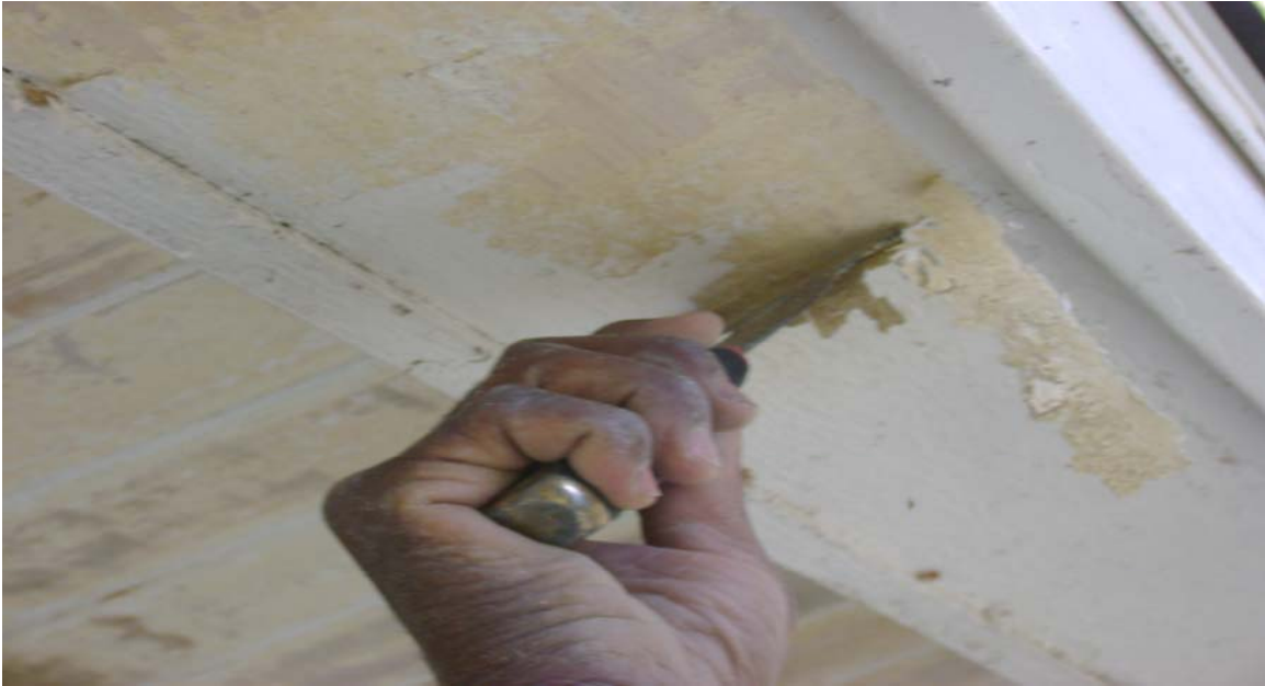
Step #3 Hand-scraping the loosened paint off the surface with a multi-purpose tool.
