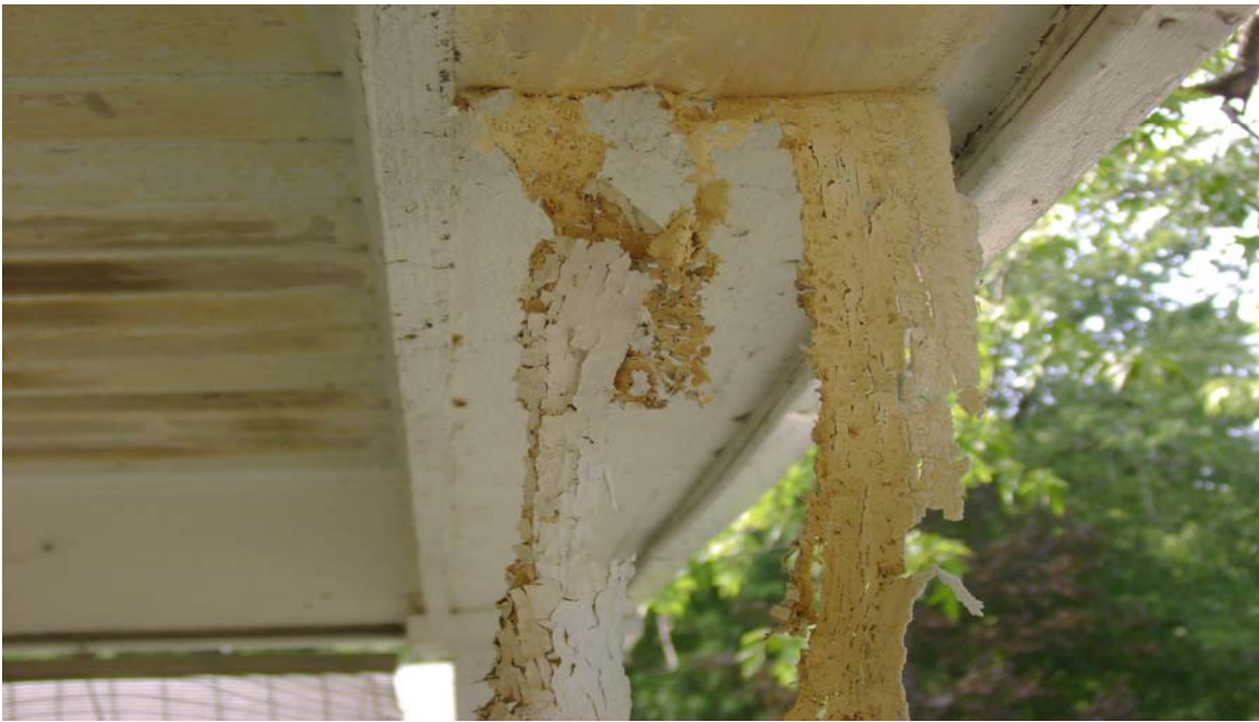
Step #2 Silent Paint Remover removed after 60 seconds.
