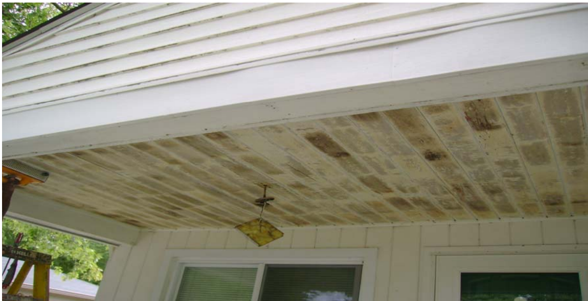
Porch ceiling after initial stripping with the Silent Paint Remover.
