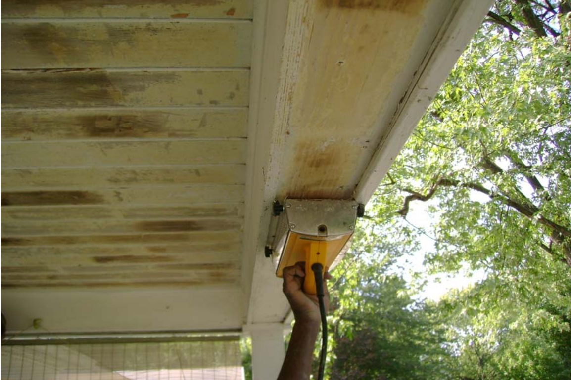
Step #1 Applying the Silent paint remover on the bottom face of the header.
