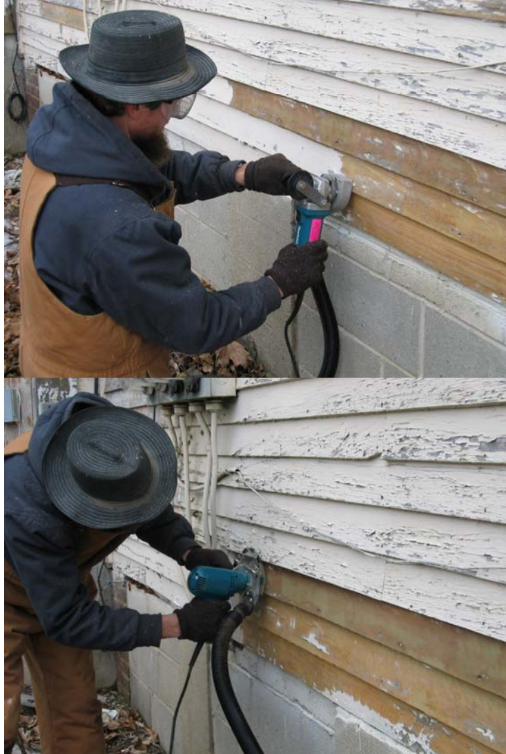
Paint Shaver® top and high-speed disc sander with suction head attachment bottom both attached to vacuum
