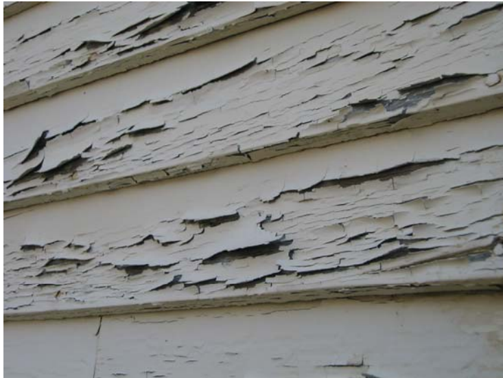
Overall view and close-up views of paint condition
