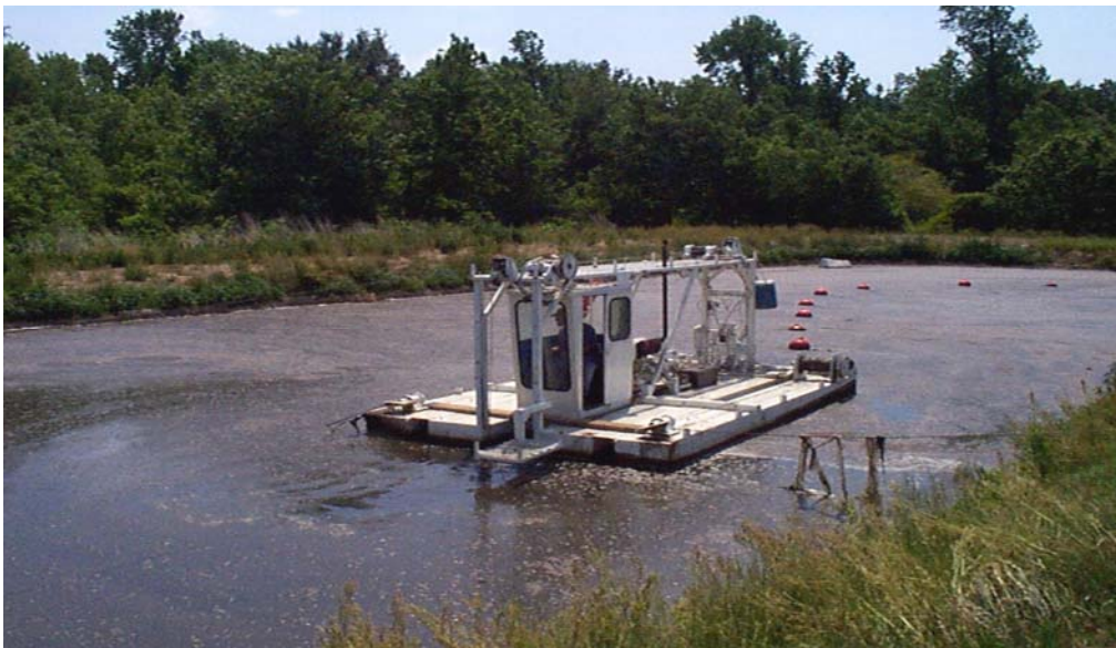
Figure 2. Pumping dredge operating in a lagoon in North Carolina.
